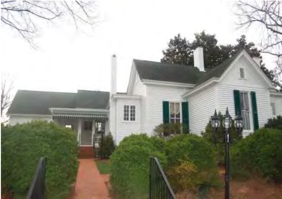
Plate 13. Reid House, Side (West) Elevation and Kitchen Wing, Looking East.
