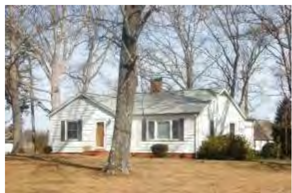
No. 92 House (PIN 07129345A), 3709 Old Monroe Road, Indian Trail, Union County
