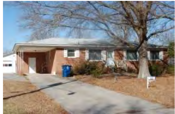
No. 45 House (PIN 07126002J), 109 Anne Street, Stallings, Union County
