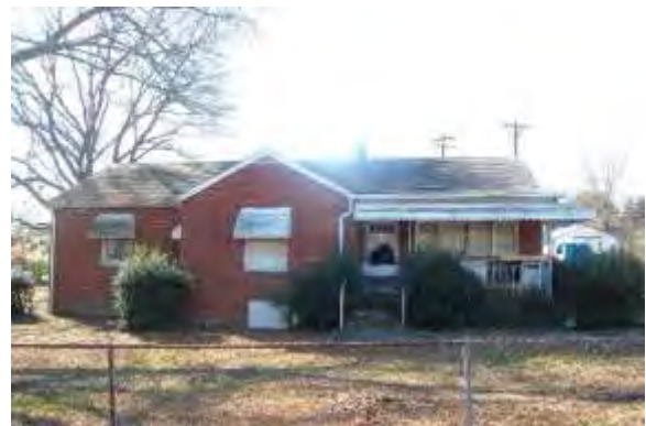
No. 53 House (PIN 07129293), 2828 Old Monroe Road, Stallings, Union County
