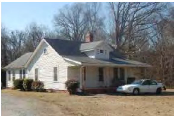
No. 59 House (PIN 07129399), 3608 Old Monroe Road, Stallings, Union County
