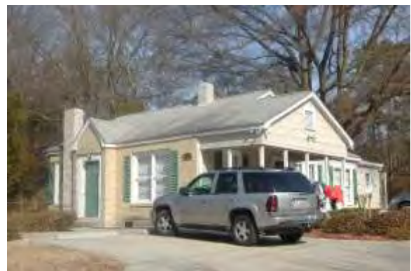
No. 90 House (PIN 07114042A), 4017 Old Monroe Road, Indian Trail, Union County
