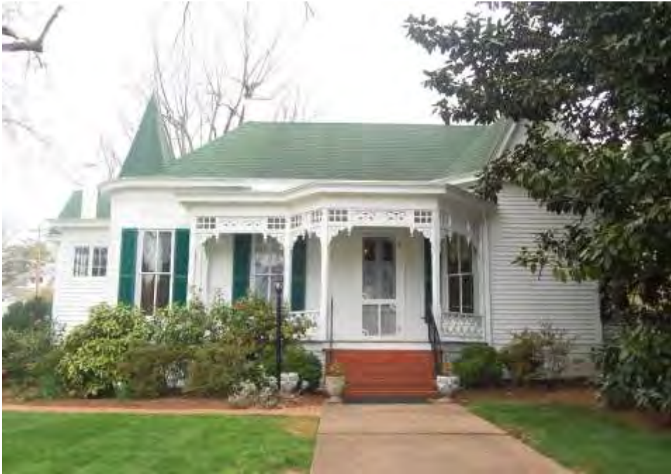
Plate 11. Reid House, House and Setting, Looking North.
