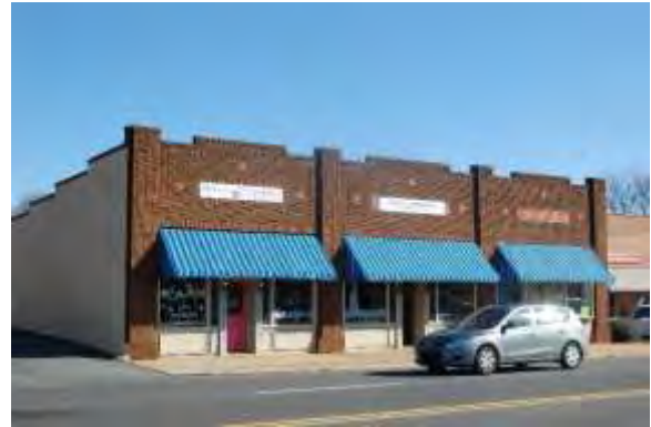
No. 4 Commercial Building (PIN 19326203), 116 West John Street, Matthews, Mecklenburg County
