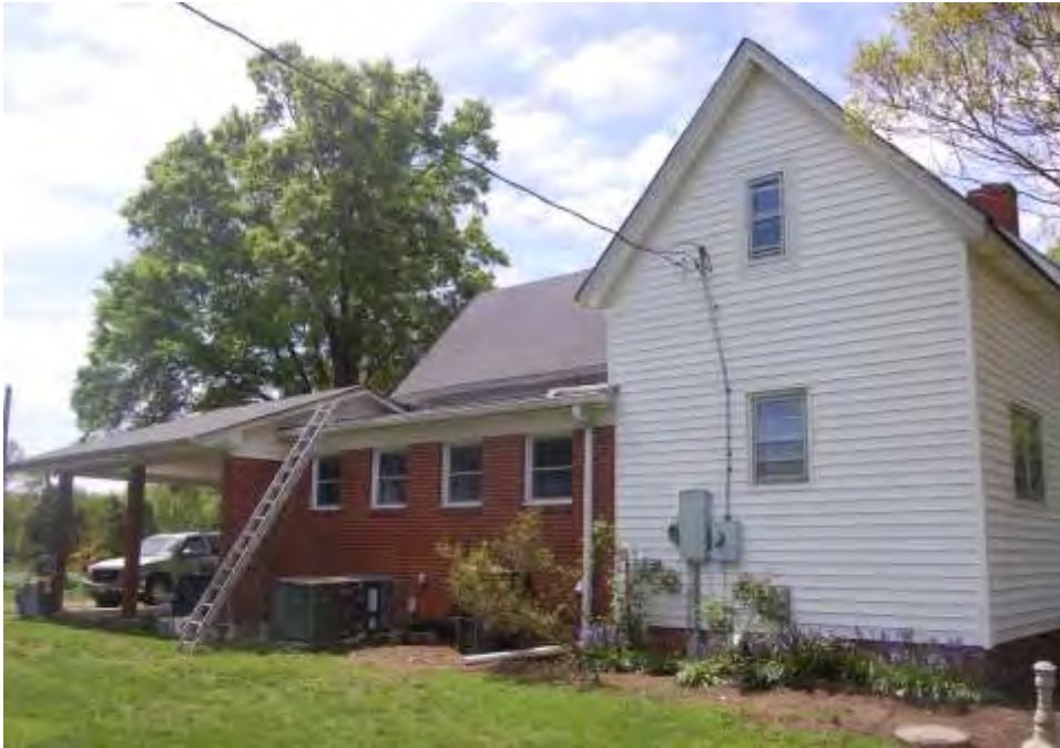
Plate 63. Heywood-Killough House, Rear (North) Elevation, Looking South.
