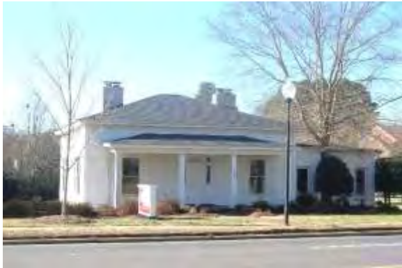
No. 2 Bain-Reid House (MK1173) (PIN 22702423), 135 West John Street, Matthews, Mecklenburg County
