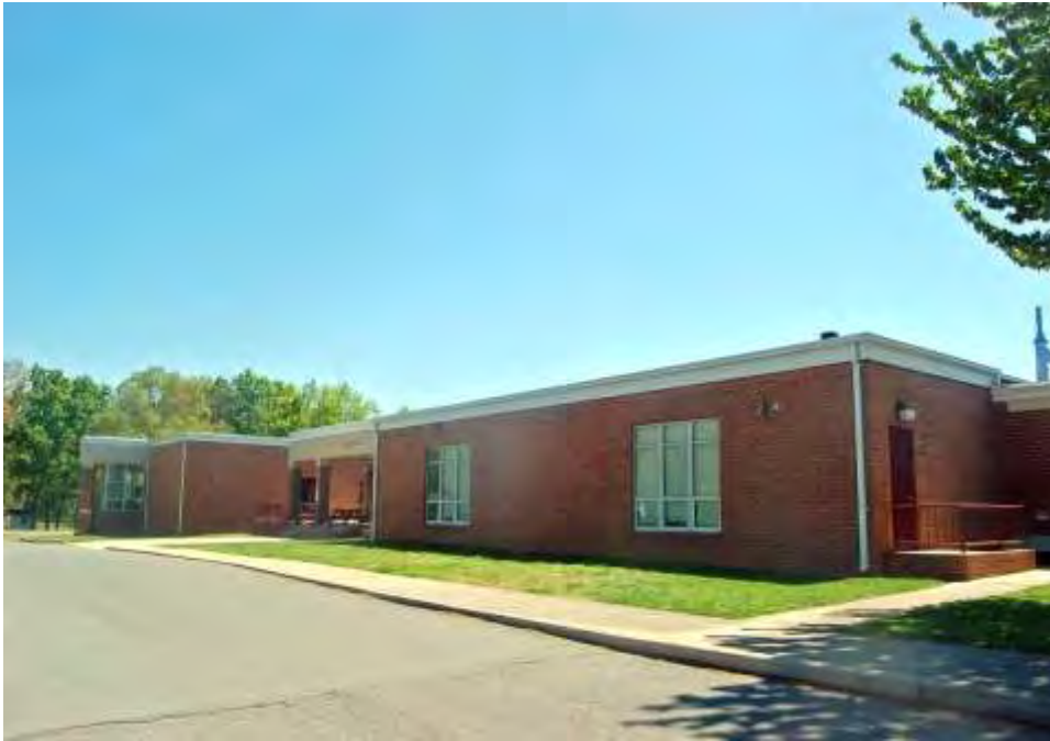
Plate 46. Sun Valley High School, East Side of North Elevation, 1993 Classroom Addition and 1993 Auditorium Additions, Looking Southeast.
