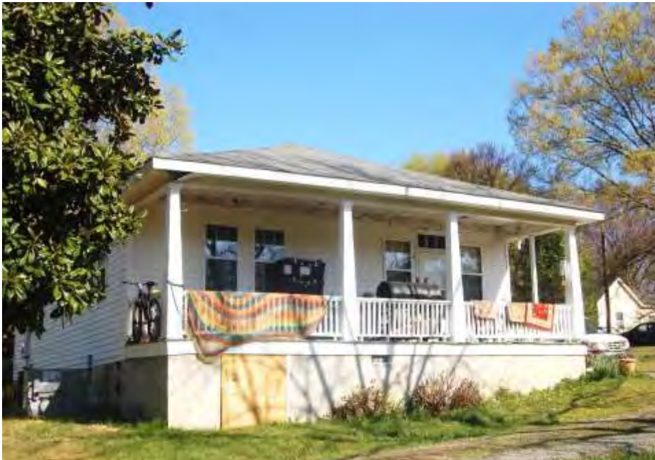
Plate 30. Crestdale, Surviving 1900s House, 617 Matthews Chapel Road, Looking West.
