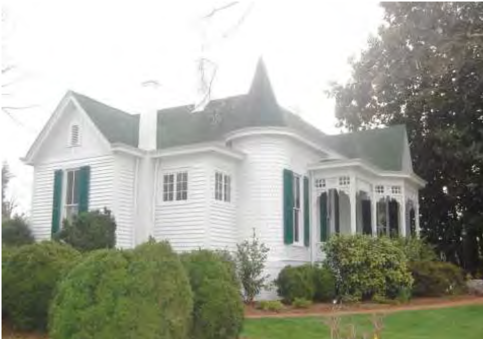
Plate 12. Reid House, Front (South) and Side (West) Elevations, Looking Northeast.
