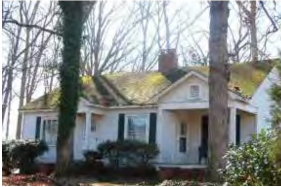
No. 29 Duplex (PIN 21501408), 352 East Charles Street, Matthews, Mecklenburg County
