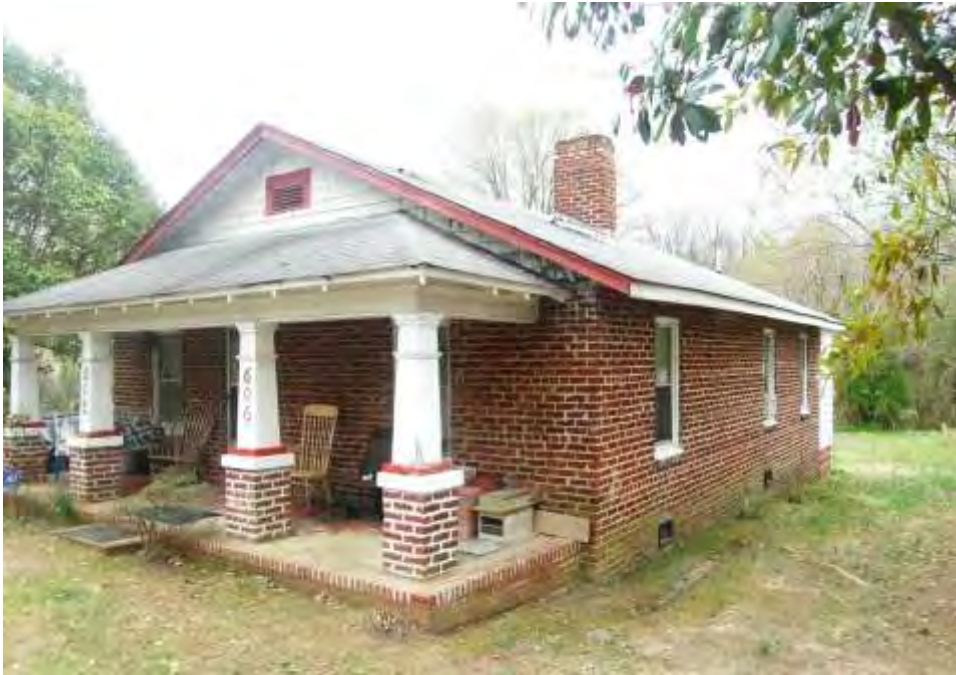
Plate 21. Rowland-Clay House, Façade and Side (West) Elevation, Looking Southeast.
