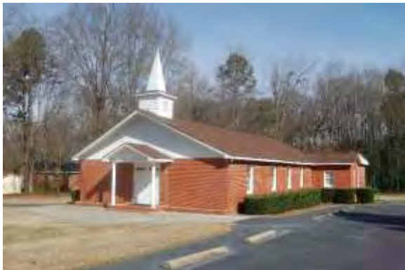
No. 83 Grace Baptist Church (PIN 07087013), 5739 Old Monroe Road, Indian Trail, Union County
