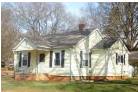
No. 91 House (PIN 07114041A), 4009 Old Monroe Road, Indian Trail, Union County
