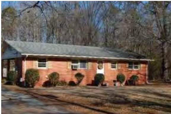
No. 57 House (PIN 07129296C), 3927 Pleasant Plains Road, Stallings, Union County
