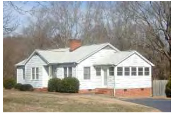
No. 94 House (PIN 07129343), 3309 Old Monroe Road, Stallings, Union County
