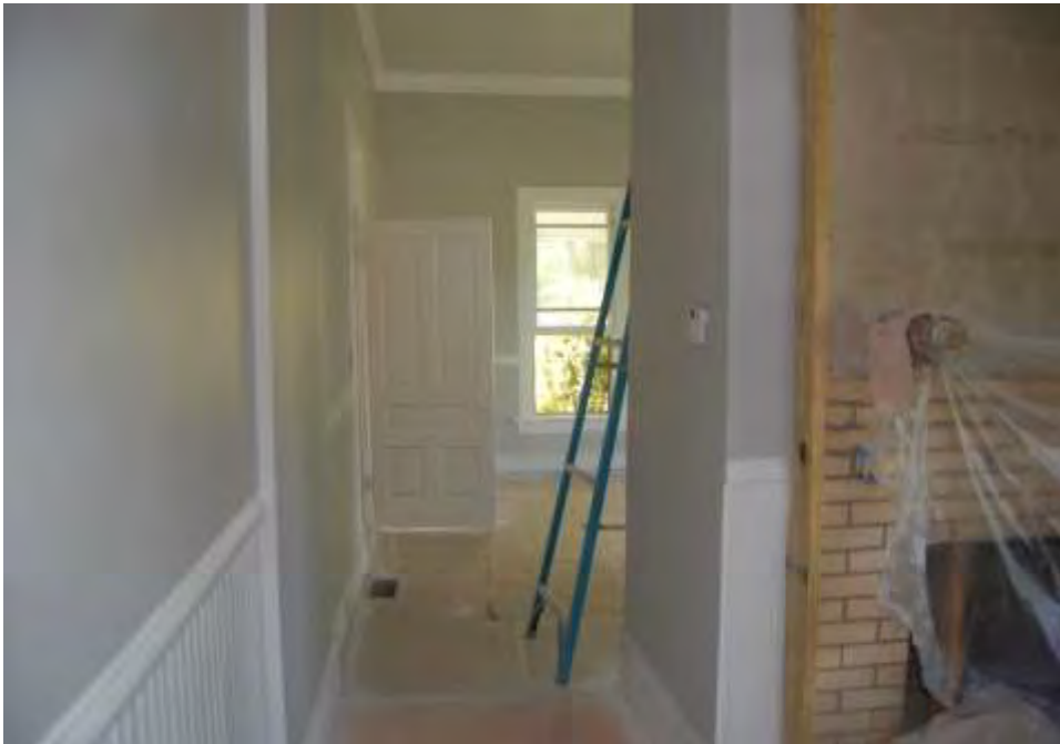
Plate 68. Heywood-Killough House, Interior, Looking South from Dining Room into Living Room.
