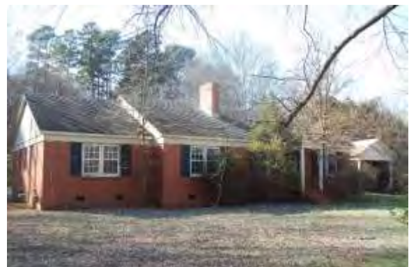
No. 66 House (PIN 07114038A), 4208 Old Monroe Road, Indian Trail, Union County
