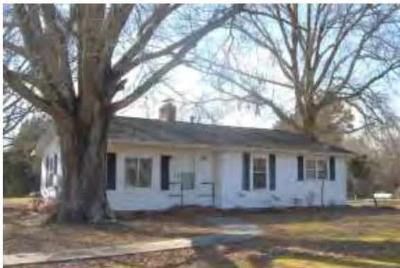
No. 71 House (PIN 07114006A), 5124 Old Monroe Road, Indian Trail, Union County
