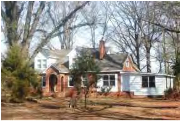
No. 85 House (PIN 07087017A), 5309 Old Monroe Road, Indian Trail, Union County
