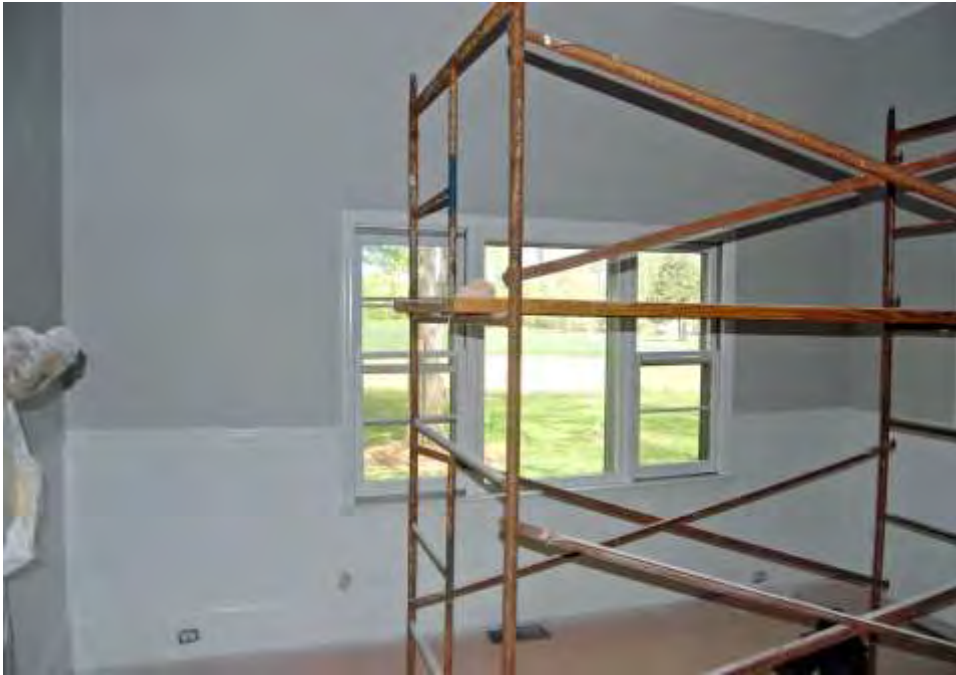
Plate 67. Heywood-Killough House, Interior, Dining Room, Added Circa 1960 Window.
