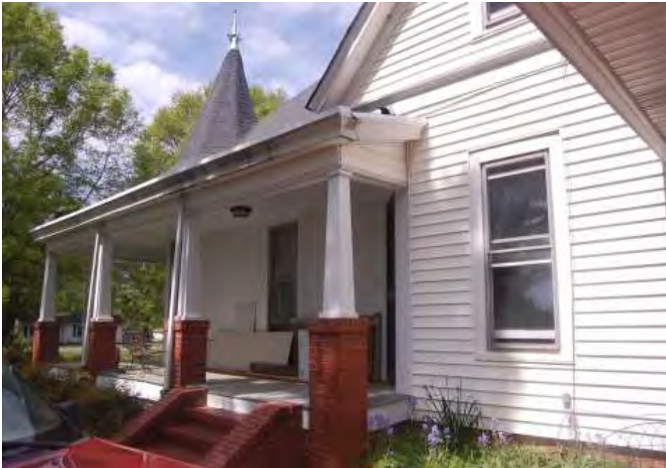
Plate 60. Heywood-Killough House, Side (East) Elevation, Looking Southwest.
