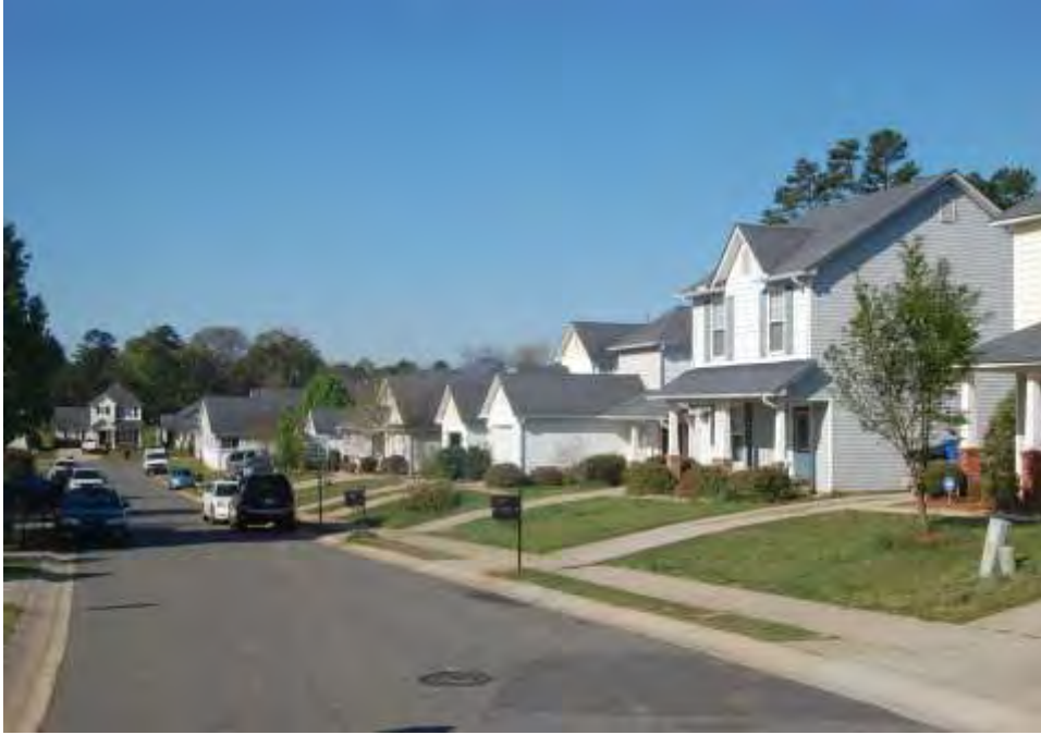
Plate 27. Crestdale, Modern Crestdale Crossing Subdivision, Looking South.
