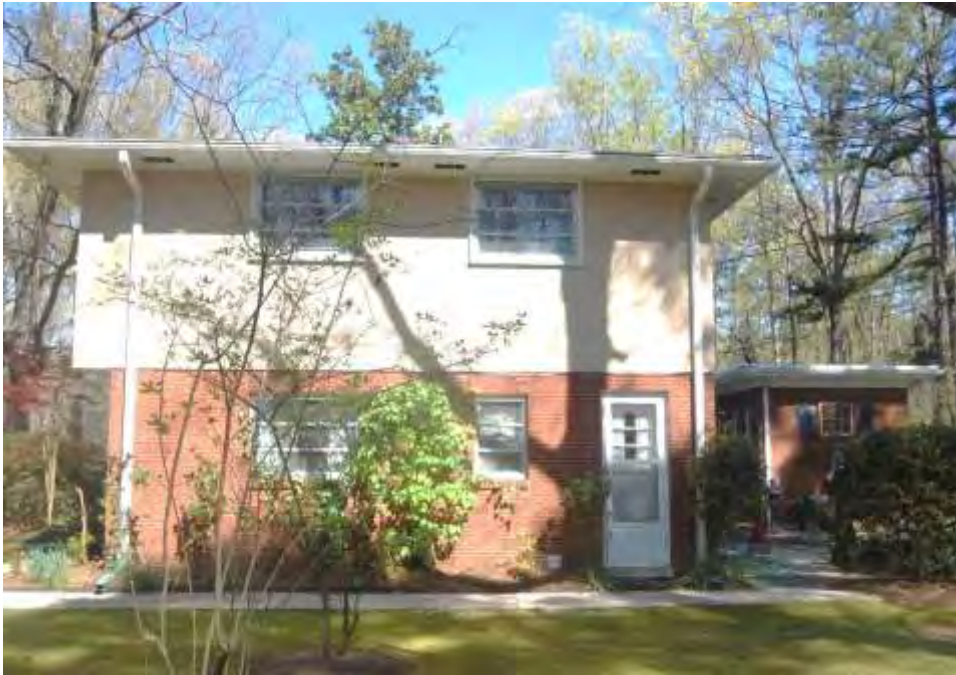
Plate 80. Banks and Carolyn Funderburk House, Side (Southeast) Elevation, Looking Northwest.
