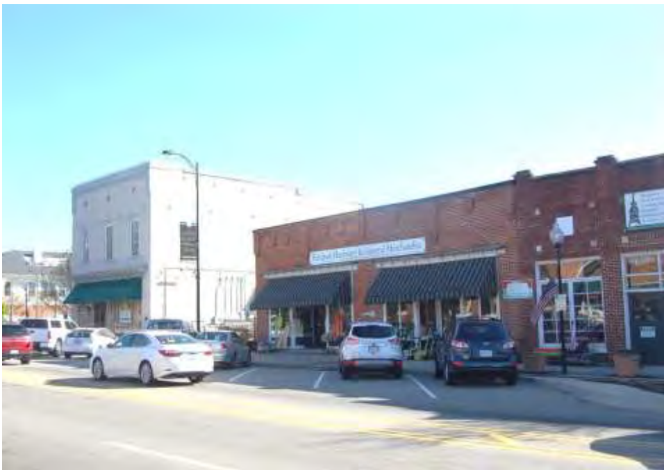
Plate 3. Matthews Commercial Historic District, Heath and Reid General Store (Left) and Renfrow Hardware Store, Looking Northeast.
