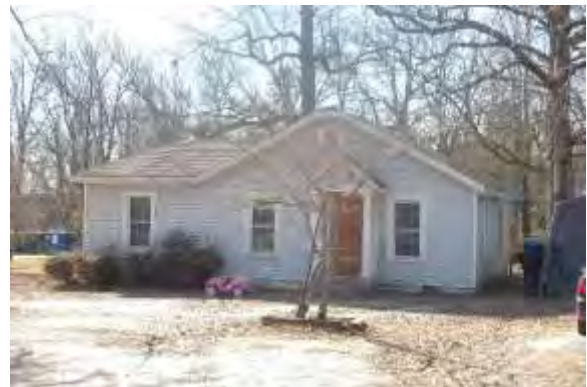
No. 51 House (PIN 07129313), 2612 Old Monroe Road, Stallings, Union County
