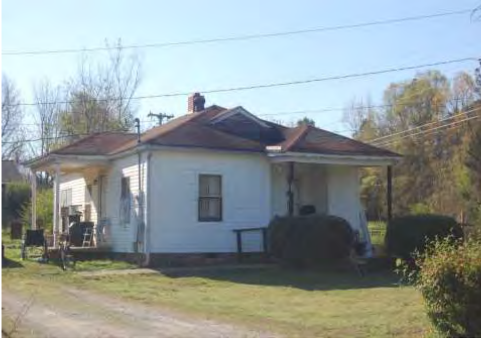
Plate 29. Crestdale, Surviving 1930s House, 318 Crestdale Road (Main Street), Looking East.
