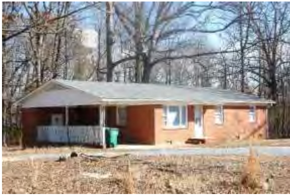
No. 48 House (PIN 07126004), 2609 Old Monroe Road, Stallings, Union County
