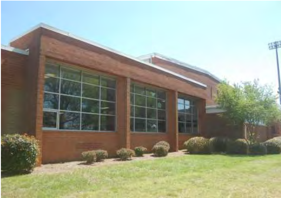
Plate 50. Sun Valley High School, 1960 Cafeteria, Replacement Windows, Looking Southeast.
