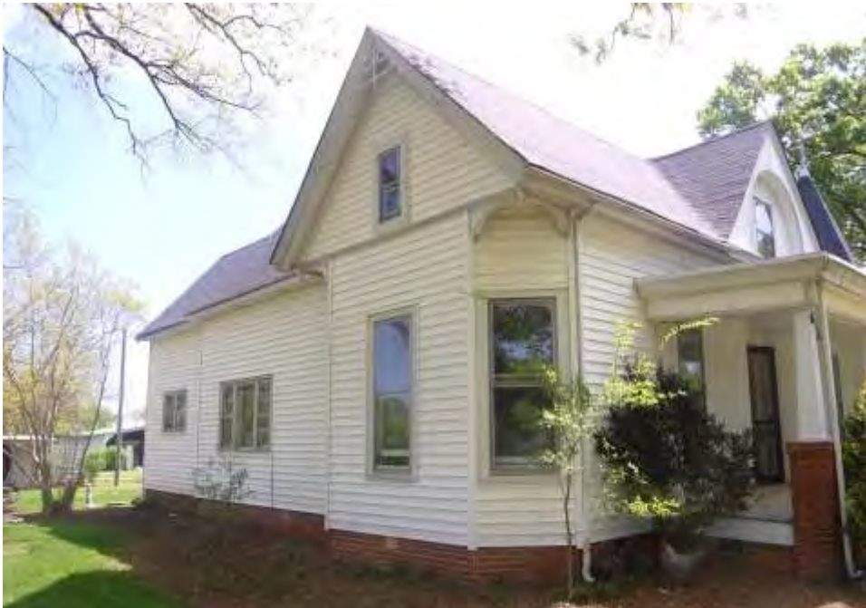
Plate 64. Heywood-Killough House, Side (West) Elevation, Looking Northeast.
