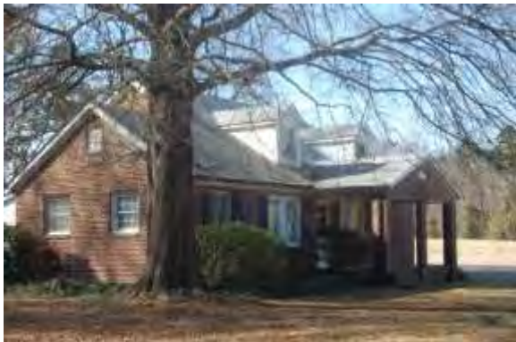
No. 65 House (PIN 07132030A), 4132 Old Monroe Road, Indian Trail, Union County
