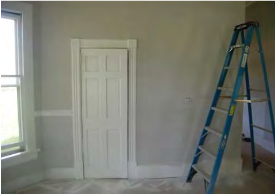
Plate 69. Heywood-Killough House, Interior, Living Room, Mantel Originally Located Right of Closet Door, Now Removed and Wall Sheetrocked.
