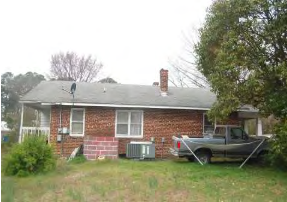
Plate 23. Rowland-Clay House, Side (East) Elevation, Looking West.
