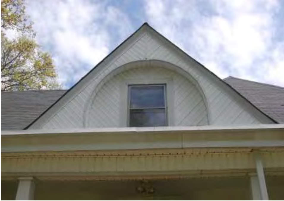
Plate 59. Heywood-Killough House, Front Gable, Looking North.
