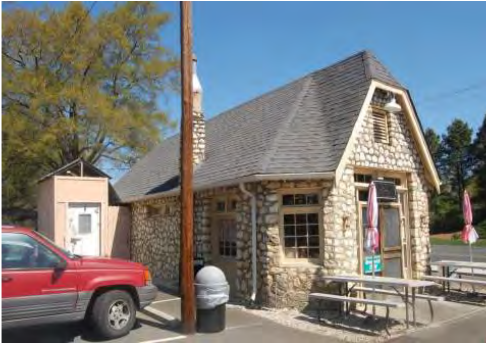
Plate 33. Banks H. Funderburk Store, Entrance and Side (West) Elevation, Looking Northwest.
