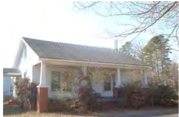
No. 64 House (PIN 07132036), 135 Chestnut Lane, Indian Trail, Union County
