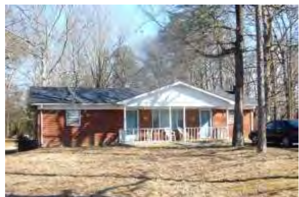
No. 47 House (PIN 07126003), 2601 Old Monroe Road, Stallings, Union County
