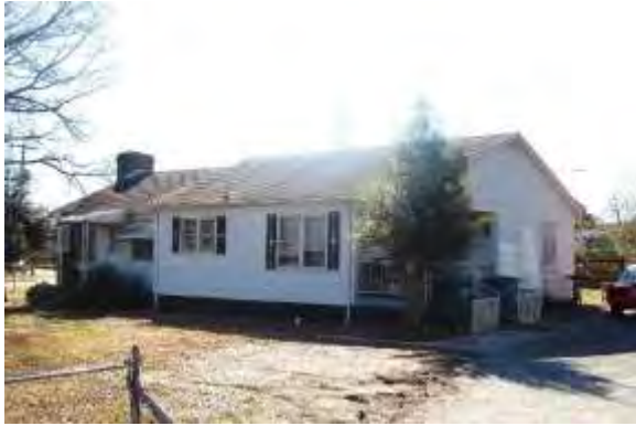
No. 54 House (PIN 07129293), 2900 Old Monroe Road, Stallings, Union County
