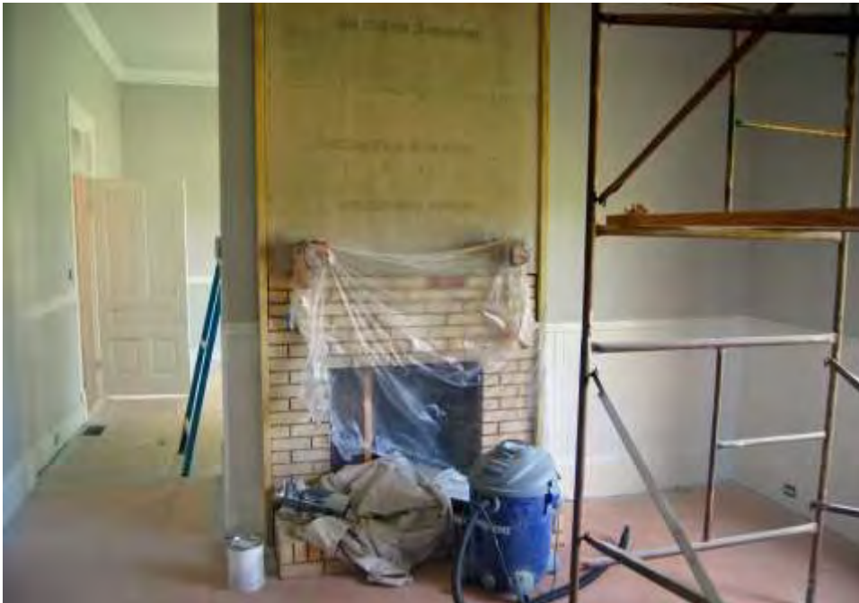
Plate 66. Heywood-Killough House, Interior, Dining Room, Fireplace.
