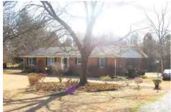
No. 70 House (PIN 07114007A), 5024 Old Monroe Road, Indian Trail, Union County
